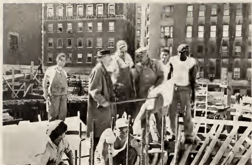
Above: Fig. 65. Frank Lloyd Wright with workers at the construction site of the museum, ca. 1956.
